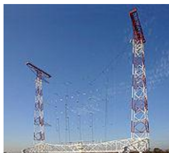
Short Wave " Curtain " Antenna (Moosbrunn, Austria)
