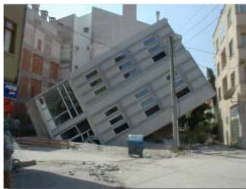
Figure: 3 Effect of liquefaction during 1999 Izmit earthquake, Turkey (S:1).
