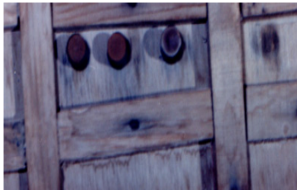
Figure 3. Photograph of untreated steel specimens after a month of atmospheric exposure.
