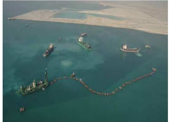
Fig. 9. Dredgers at work in front of the reclamation area.
