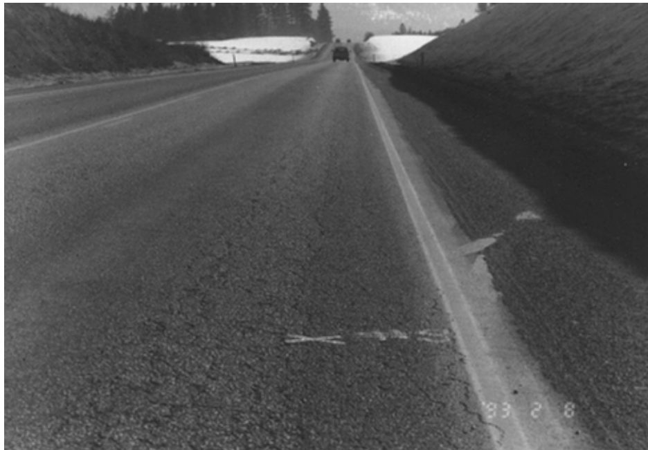
Photo 10. MP 209.40, NB lane, alligator cracking, which occurs in both wheel paths
