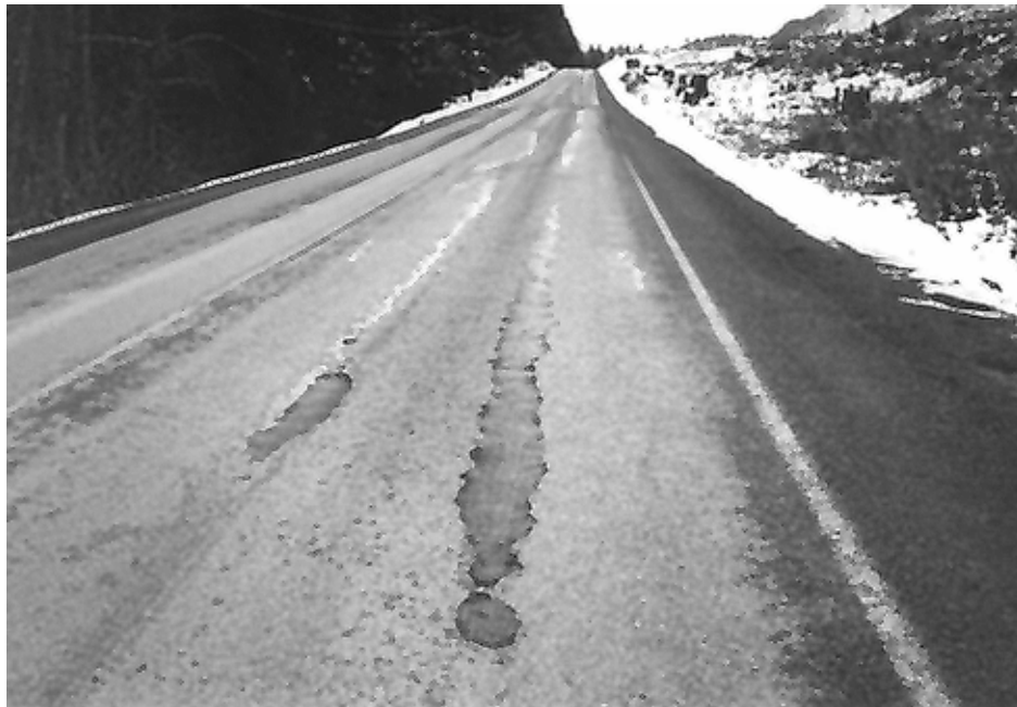
Photo 11. MP 15.08 NB, Maintenance has placed several HMA or BST patches
