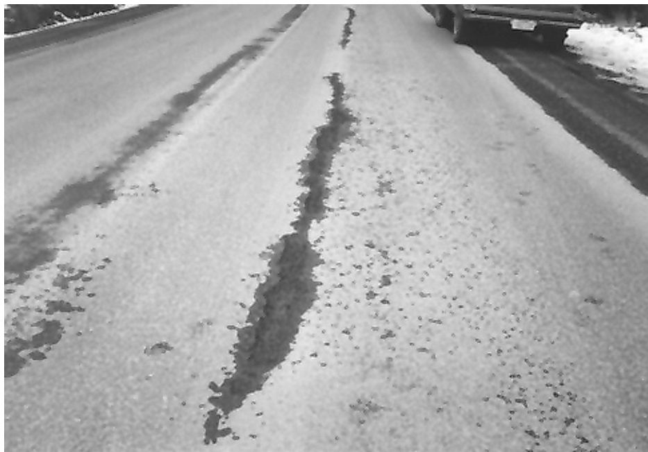
Photo 10. MP 9.98 NB, location of wide longitudinal cracking. Damage may be caused by snowplows
