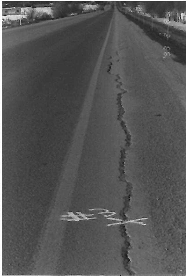
Photo 2. MP 208.00, NB shoulder cracking, occurring from MP 207.82 to MP 208.29
