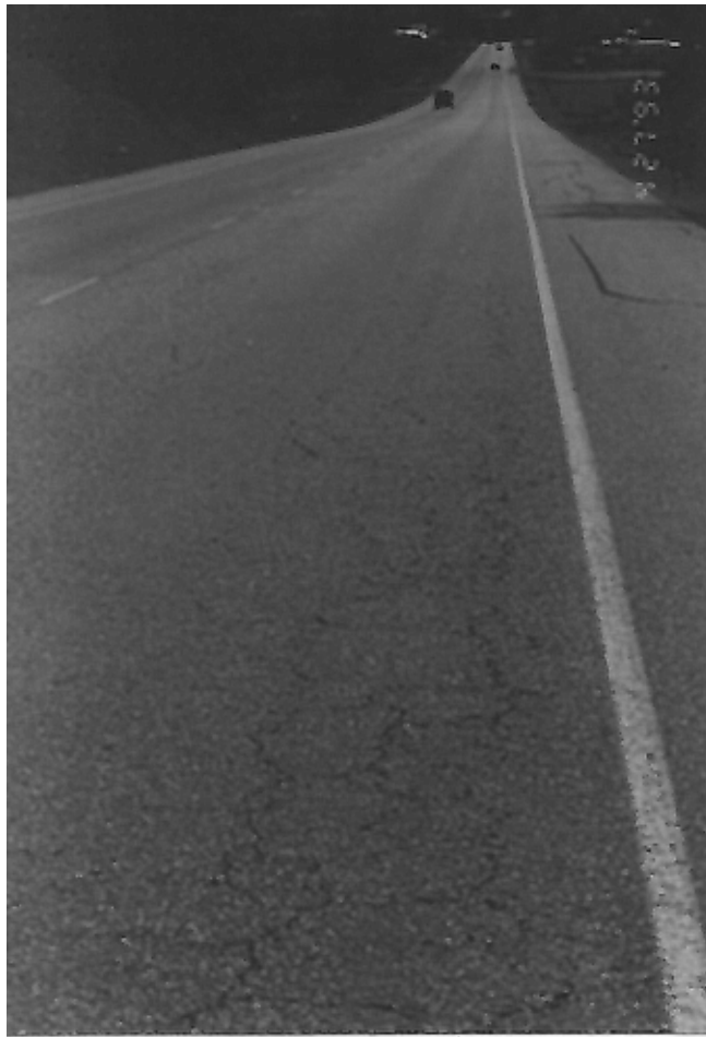
Photo 5. MP 208.56, NB lane, typical alligator cracking within the wheel paths
