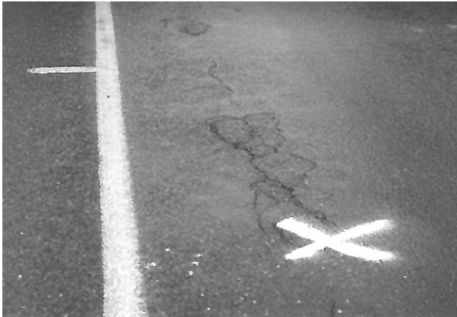
Photo 8. MP 7.18 SB, pavement has several maintenance patches and rutting
