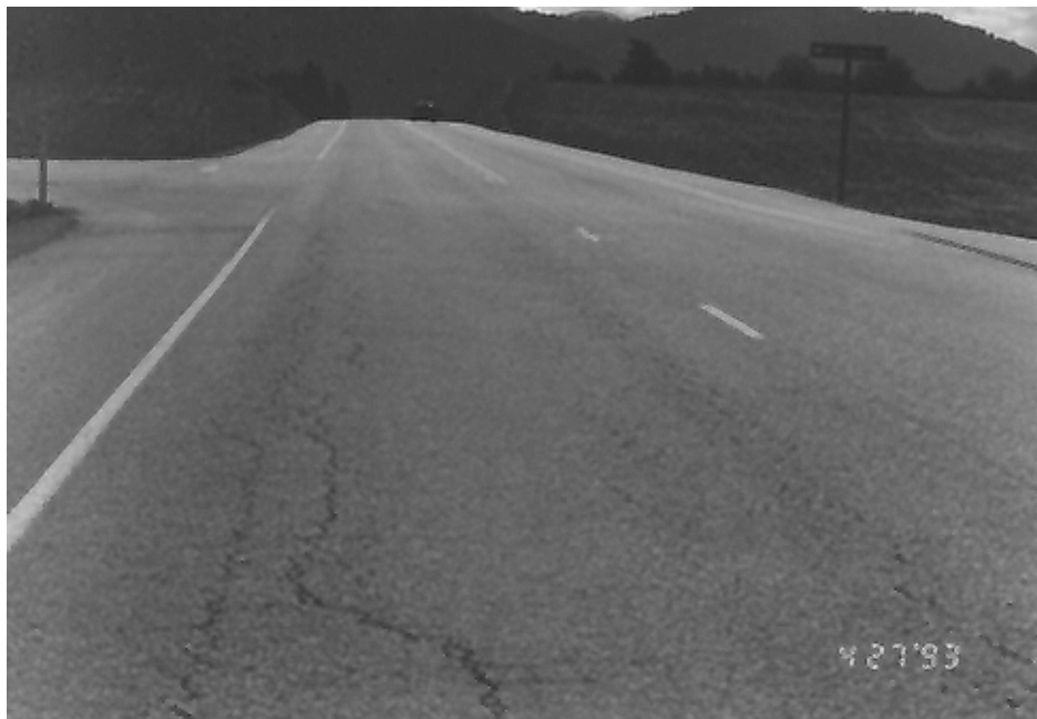
Photo 11. MP 209.60, NB lane, alligator and longitudinal cracking
