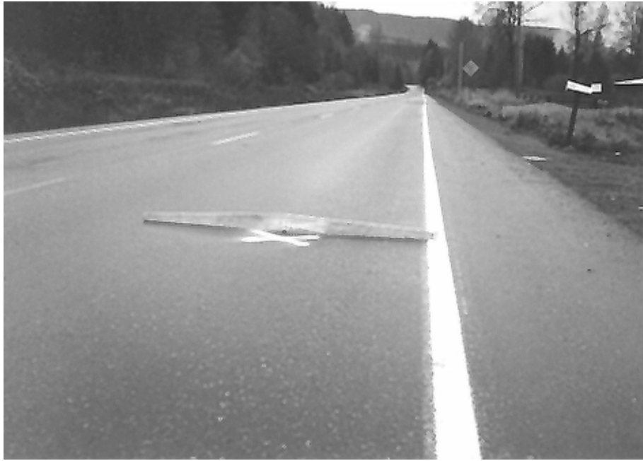
Photo 5. MP 2.83 SB, pavement in relatively good condition, pavement rutting is present
