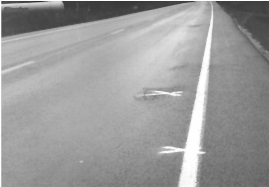
Photo 6. MP 3.68 NB, core taken at localized pavement distress
