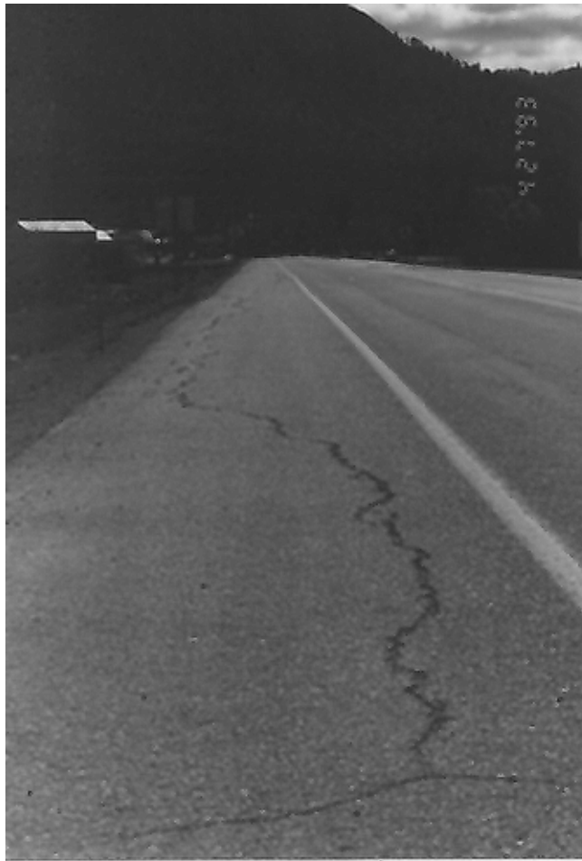
Photo 3. MP 208.07, cracking within the NB shoulder
