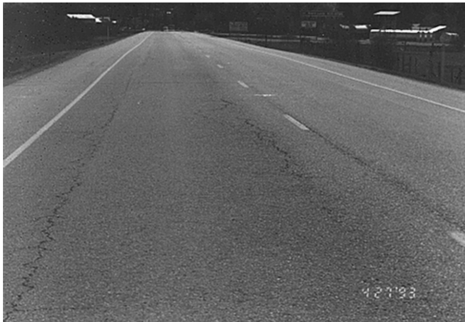
Photo 4. MP 208.18, NB lane, longitudinal cracking progressing to alligator cracks
