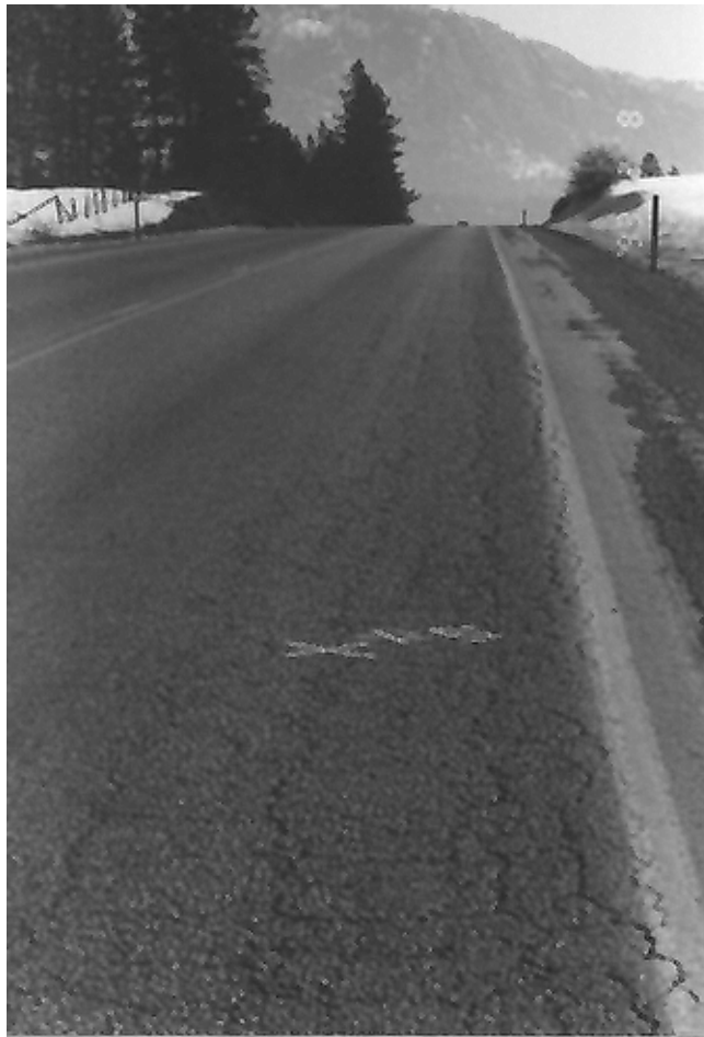
Photo 8. MP 209.00, SB lane, looking south, alligator cracking within outside wheel path
