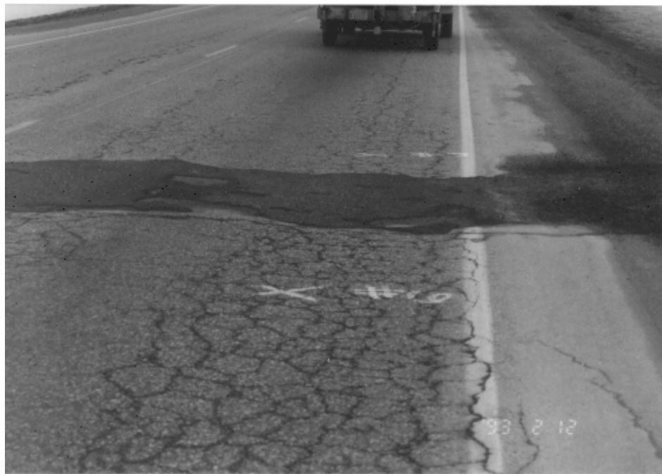
Photo 9. MP 209.05, SB lane, frost heave causing 150 to 200 mm of differential movement
