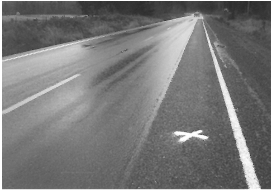
Photo 9. MP 9.96 SB, location of freeze/thaw damage, which is typical of this section for several km. Damage could be caused by snowplows and heavy truck traffic
