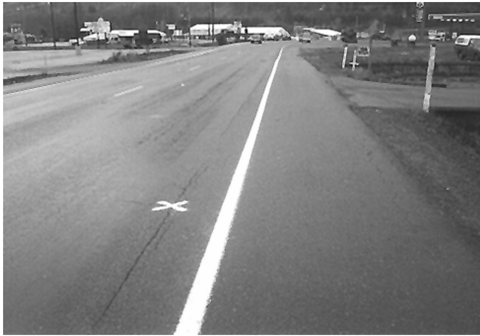
Photo 3. MP 0.44 SB, transverse cracking at the core location (marked with an "X")
