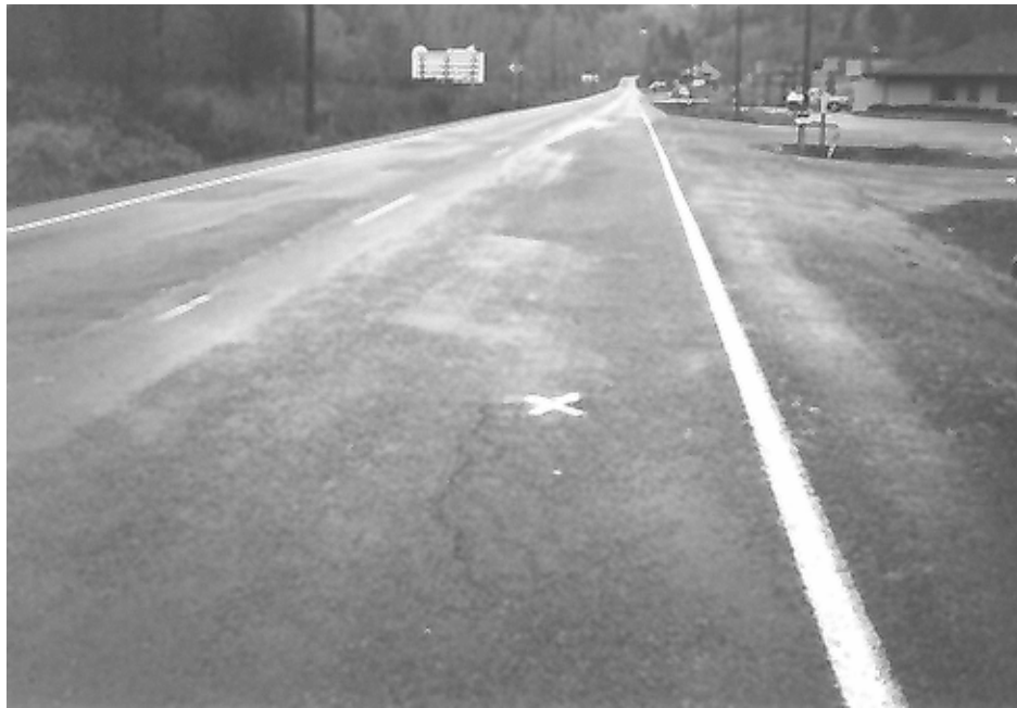
Photo 4. MP 0.99 NB, core taken at full depth longitudinal crack. This section has numerous Maintenance patches
