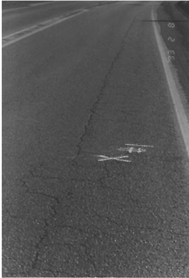
Photo 1. MP 207.90, NB lane, area of longitudinal and alligator cracking
