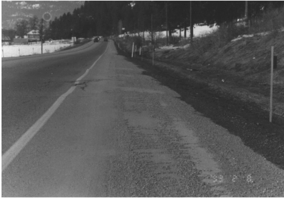
Photo 12. MP 209.82, NB lane, frost heave that affects the NB lane and shoulder
