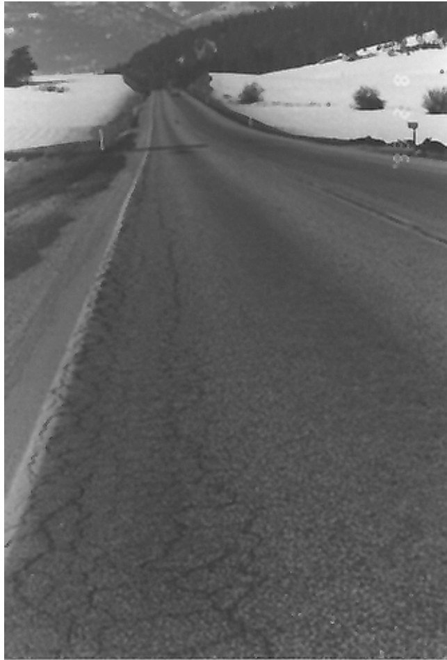
Photo 7. MP 209.00, SB lane, looking north, alligator cracking within outside wheel path
