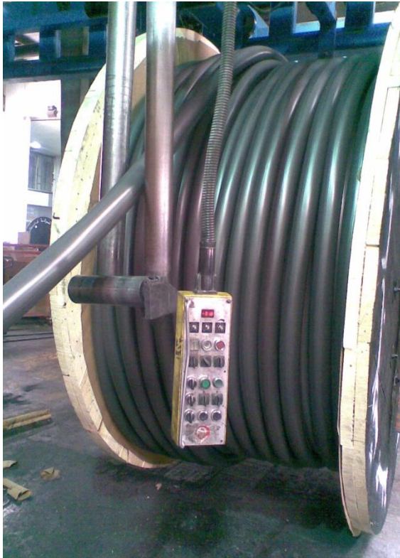
Figure 9: Cable After Bedding Stage
