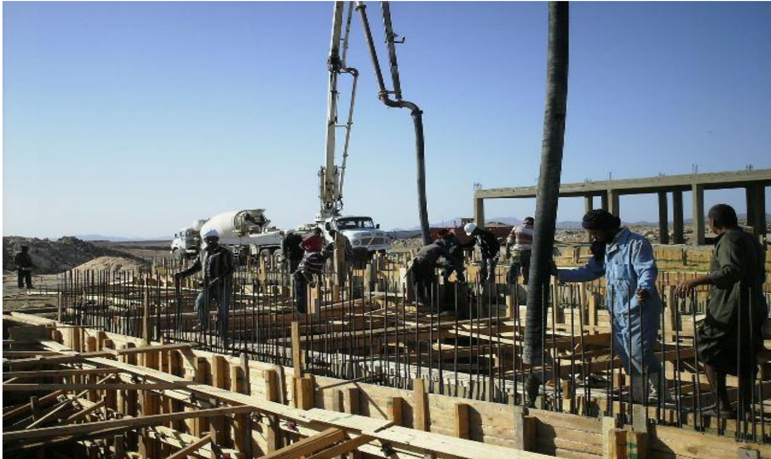
Fig: Construction Site with Labor, Materials and Equipment
