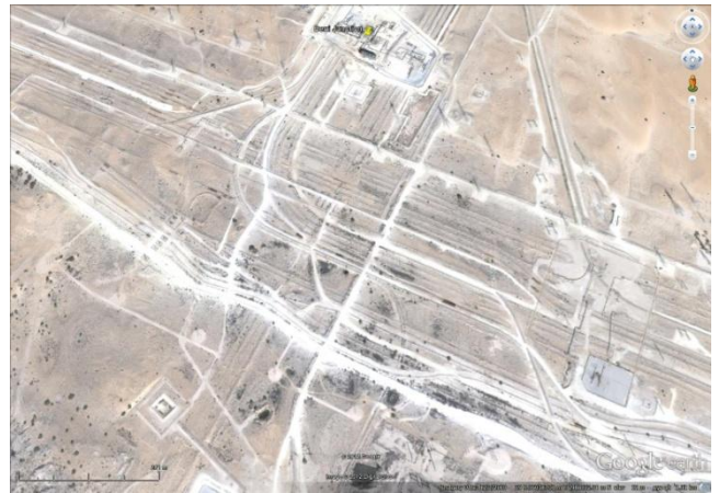
Figure 1: A map shows the congested crossing at Berri junction (source: Google Earth)
