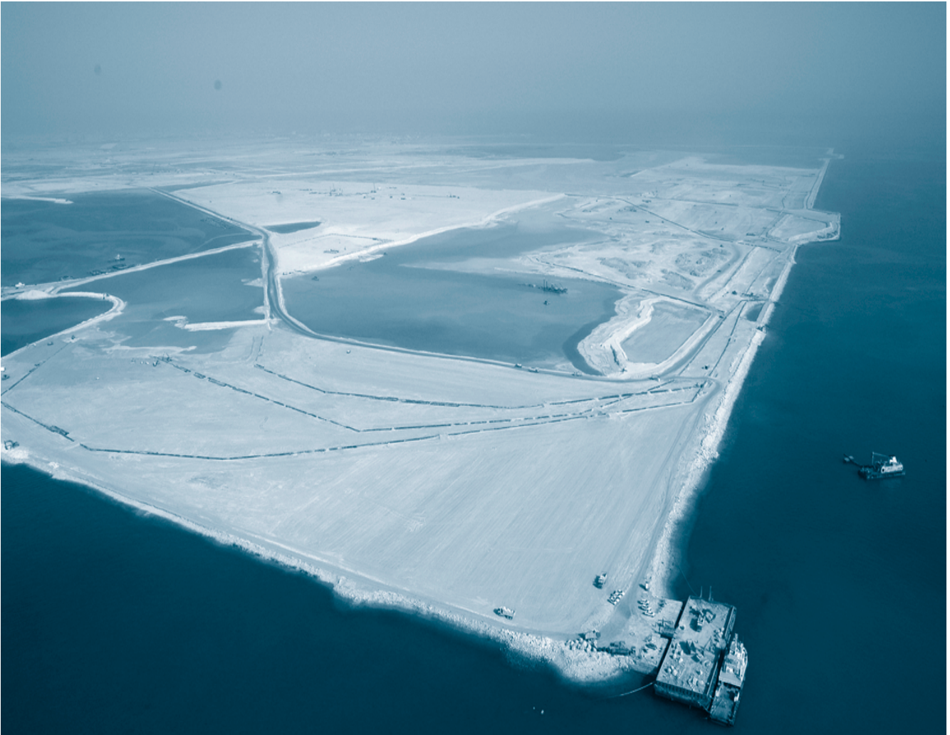
Figure 18. An aerial overview of the New Doha International Airport site. High Energy Impact Compaction with rollers was checked by the Six Sigma quality management system.
