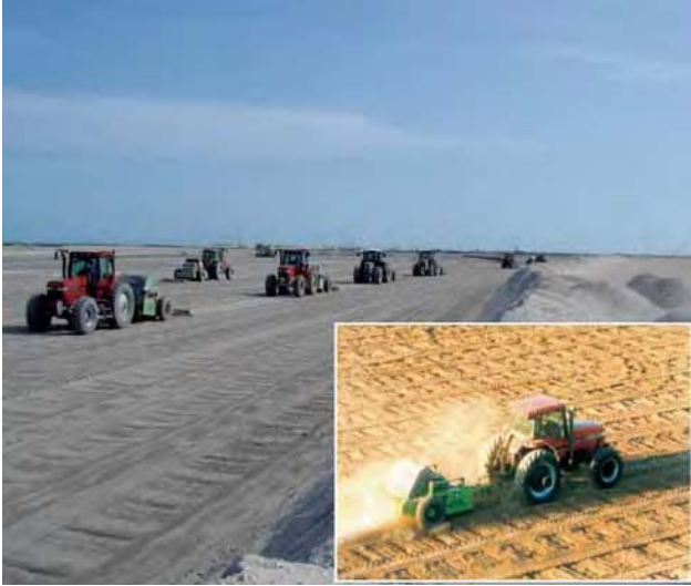
Figure 12. HEIC compactors on the NDIA project
