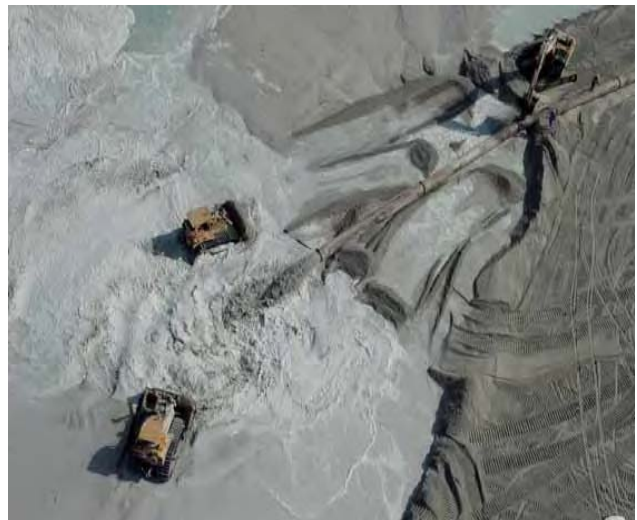
Fig. 10. Initial compaction with bulldozers in front of the discharge pipe.
