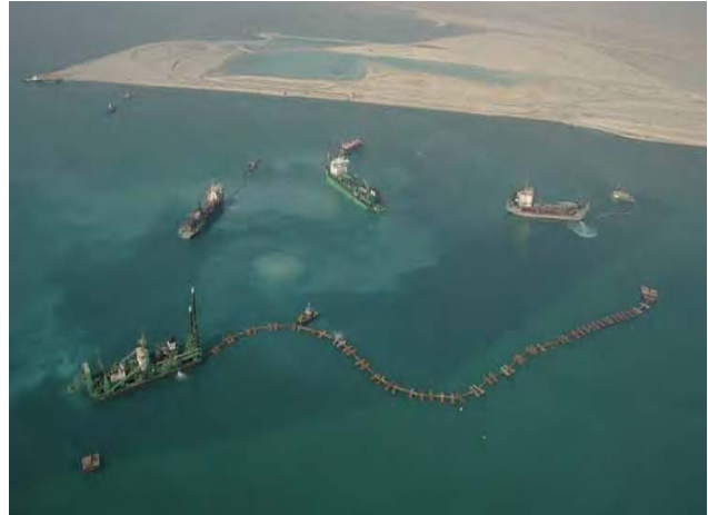
Fig. 9. Dredgers at work in front of the reclamation area.
