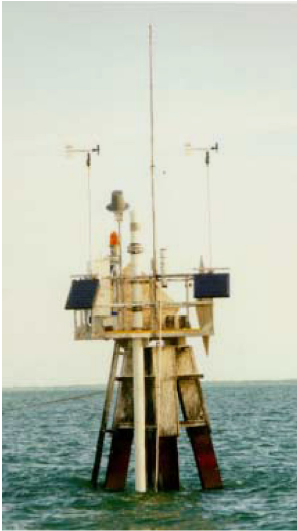
Fig. 10. Ocean observation systems as independent satellite structures. Source: Tampa Bay PORTS—University of South Florida.
