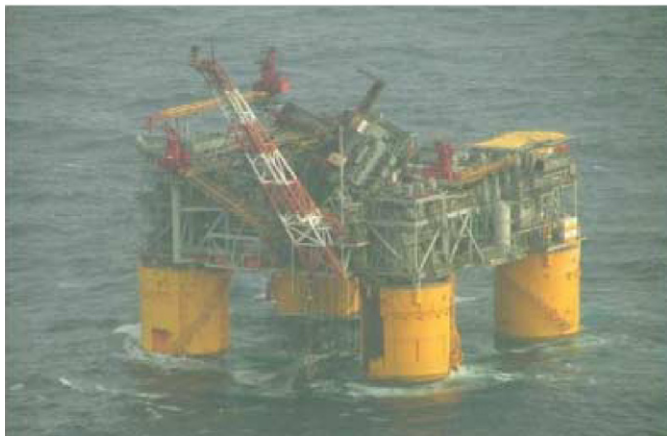
Fig. 4. Mars tension leg platform before and after Hurricane Katrina. Source: Shell.
