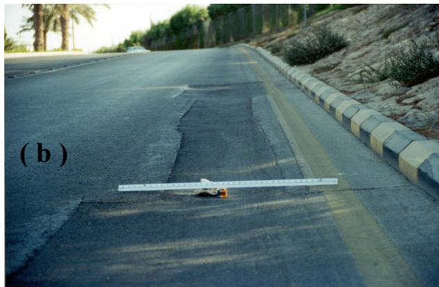
Figure 1. Typical road deterioration in the Dammam area (a) due to the use of water sensitive calcareous sediments as a graded base layer and (b) due to poor construction of utility trenches
