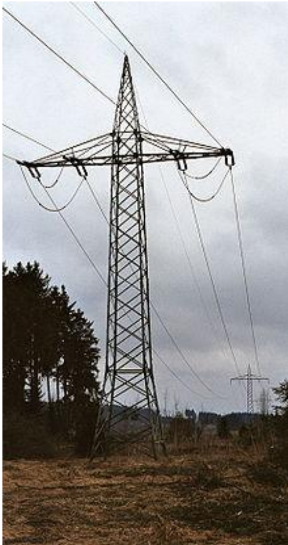
Figure: parallel overhead lines.
