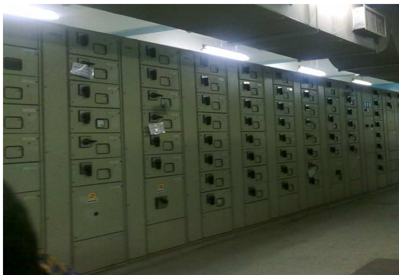
Figure 5: MCC of Finish Mill
