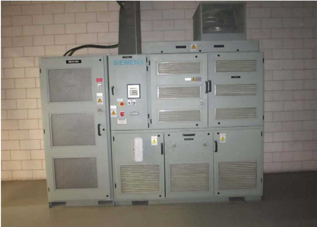
Figure 7 : VFD for motor with 1000 hp , 4160 V
