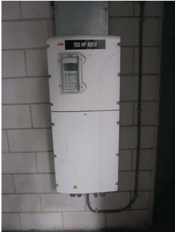
Figure 6 : VFD for motor with 100 hp , 480 V
