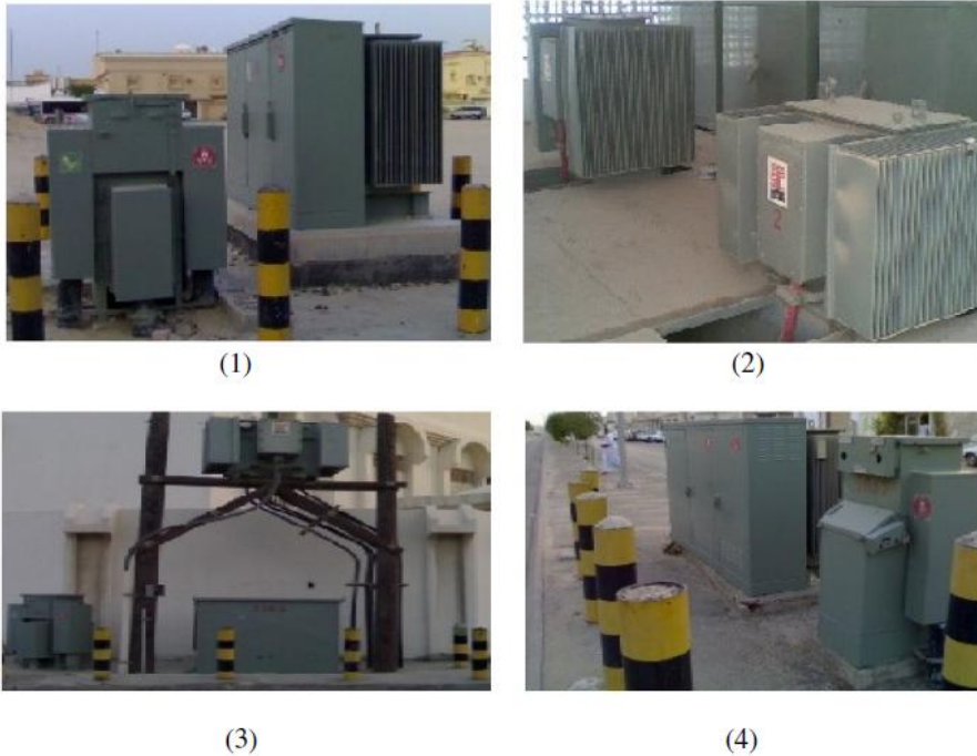
Figure 2.1: Substation types ;(1) the outdoor substation, (2) indoor substation, (3) pole mounted transformer substation, and (4) the street light substation.
