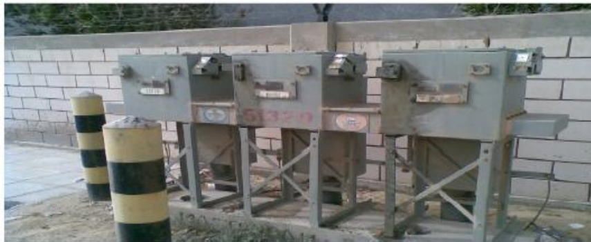
Figure 2.4: An oil switch with three legs.
