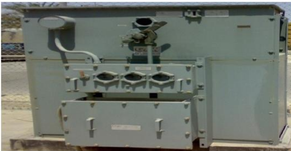
Figure 2.3: Automatic change over switch.
