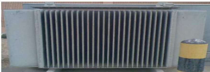
Figure 2.5: The transformer in an outdoor unit substation.
