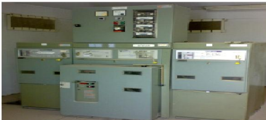
Figure 2.10: Metering unit with a multiplying factor of 13800/115.
