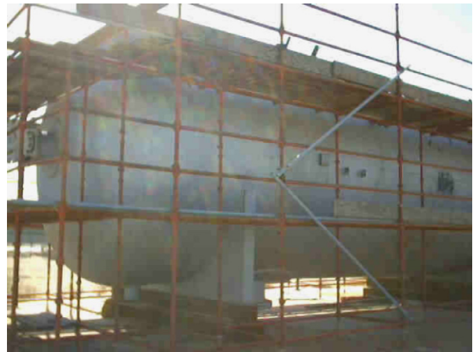
Fig. 2. Out-of-service pressure vessel used to collect the data.
