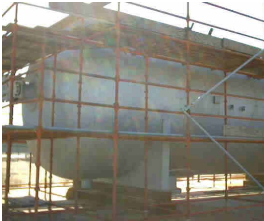
Figure 1: An out-of-service pressure vessel
