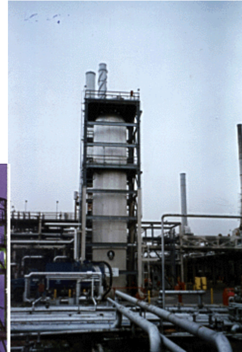
Fixed Bed Reactor
