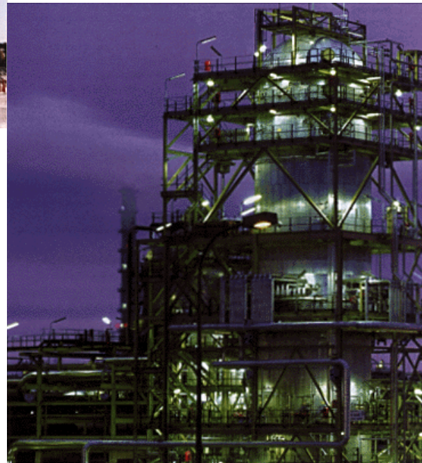
Sasol Advanced Synthol (SAS) Reactor
