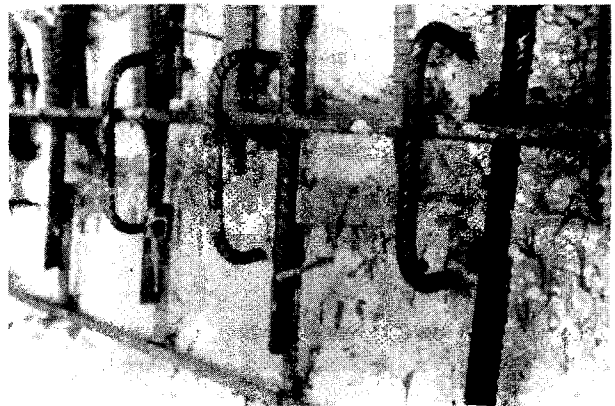
FIG. 5. Platform/Walls Joint after Installation of Stitching Dogs
