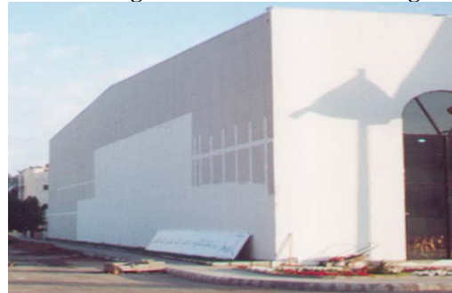
Fig 4. Cement Board Cladding
