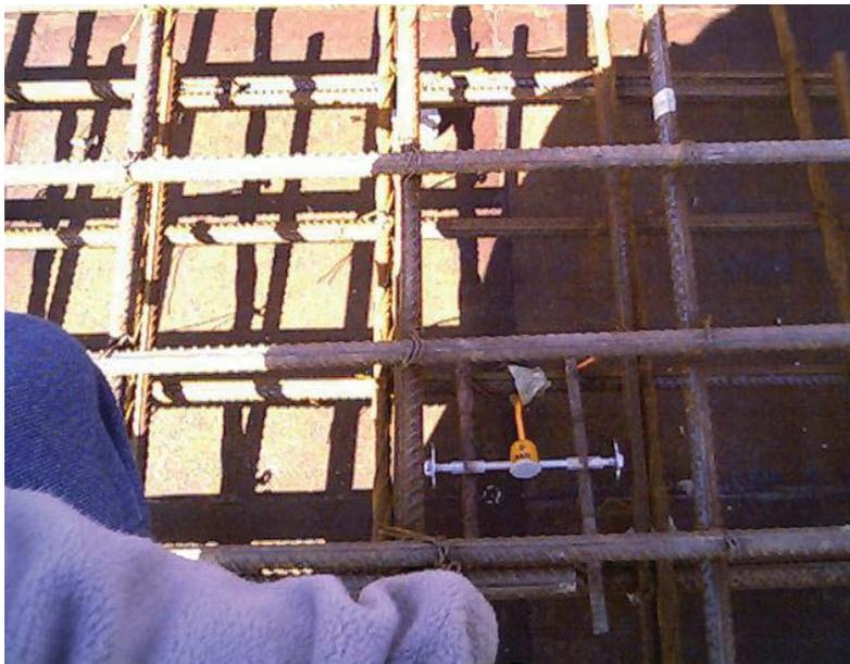
**Figure 11.** Installation of VW strain gauge
